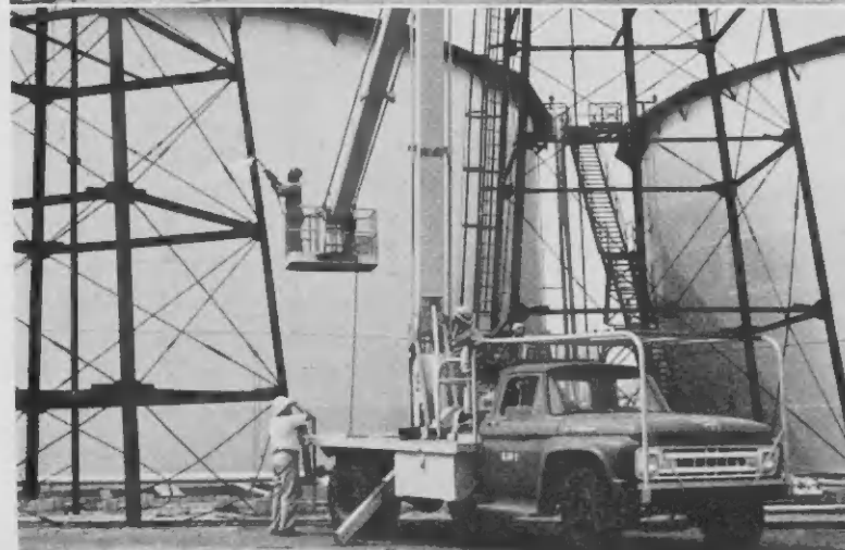
WHILE THE tall crane held the tank from above, the supporting legs were progressively cut off from below. As the legs were shortened the tank was lowered until at last it rested close to the ground where it was of such size that it could handily be placed on a truck and carted away as scrap.
